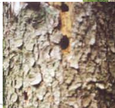
Loose bark and woodpecker damage
